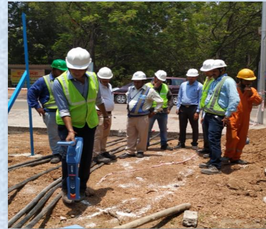
Usage of Underground Live Cable Detector and High-voltage protection gloves
