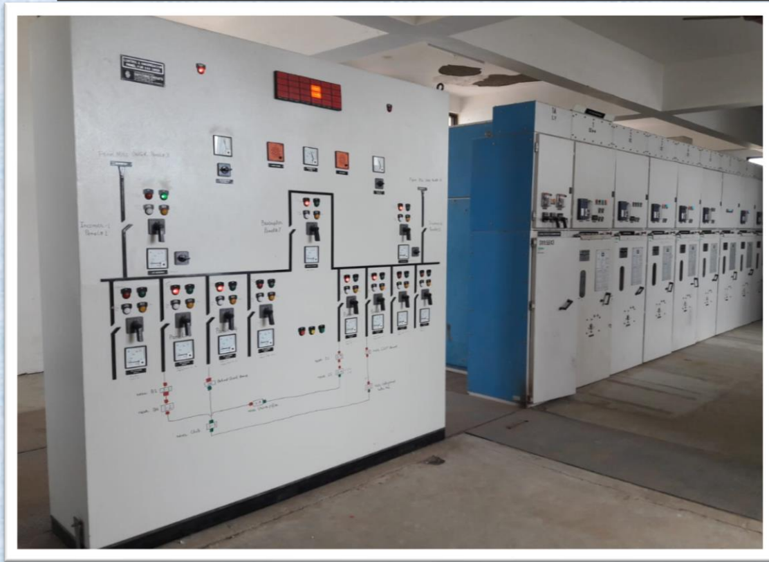
LT Package at NTPC-Gadarwara Site
