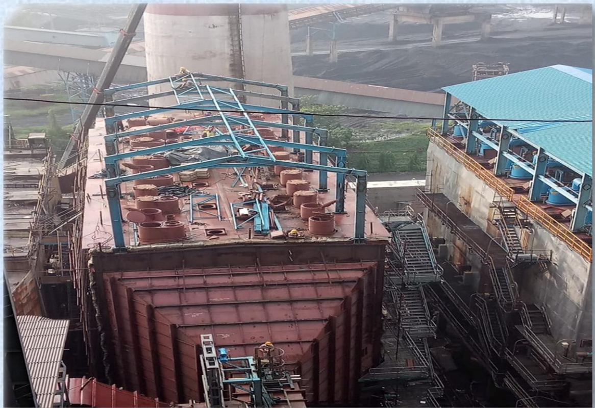
New pass erection successfully completed for NSPCL Durgapur U#1
