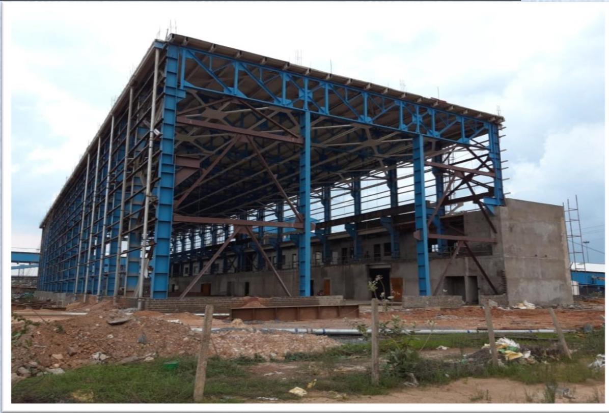
Ongoing work (Workshop Building) at NTPC-Lara site
